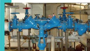
A reduced pressure principle (RP) backflow prevention device and pressure gauge.
