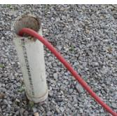
A potential backflow incident could occur at this cross-connection.
