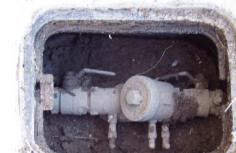
This backflow prevention device is below grade and could result in a fine.
